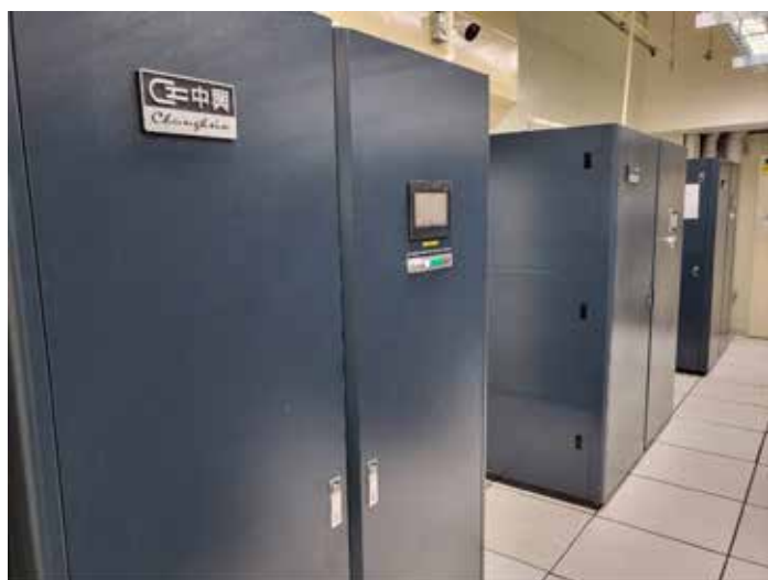
High sensible heat EC Fan constant temperature and humidity box-type unit
